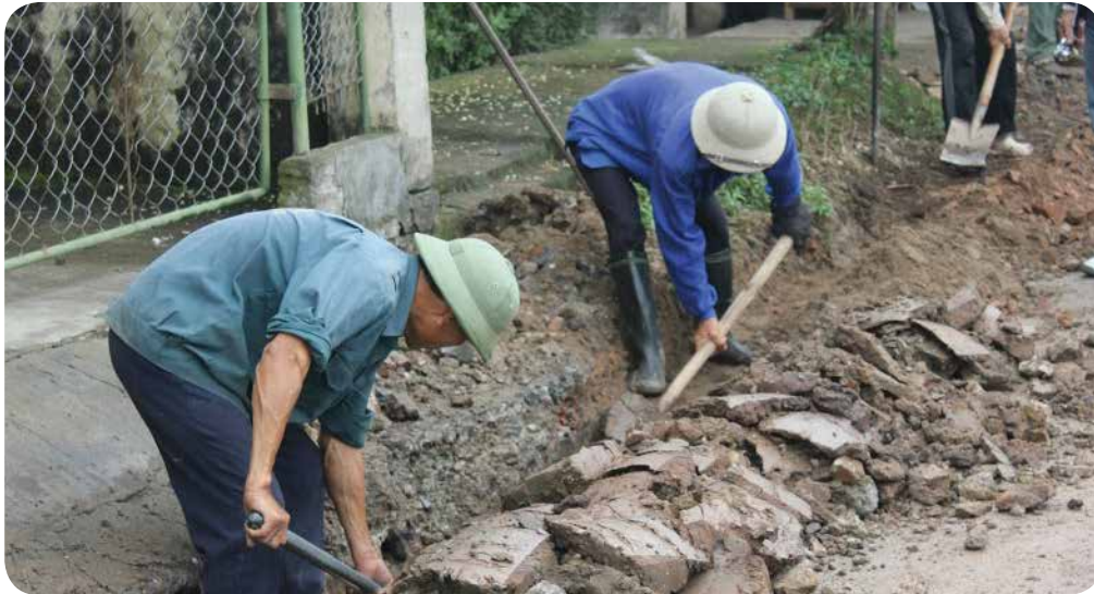
Building Water Supply Infrastructure in Rural Vietnam Habab Taifour/World Bank
